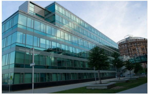
Office Campus Gasometer, Wien
